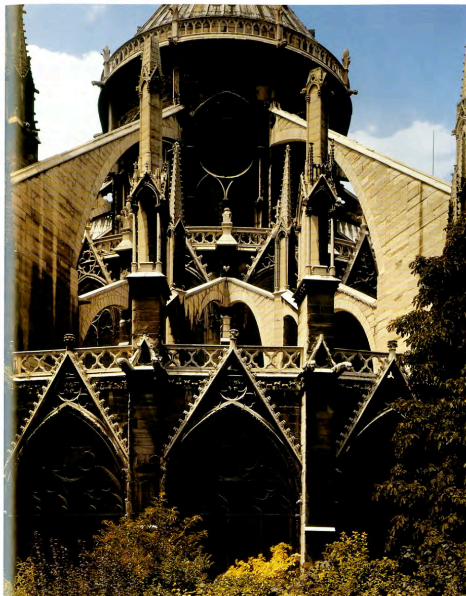
Fig. 16.12. Cathedral of Notre Dame, Paris. View of flying buttresses
