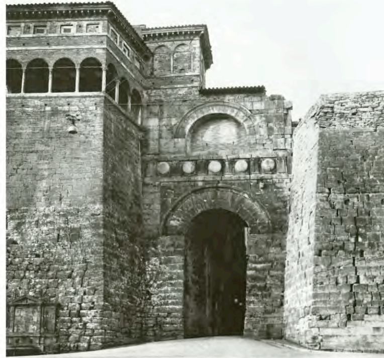
5.3 Semicircular “Arch of Augustus,” Perugia, after 310 BCE. The lower portions were constructed by the Etruscans. The Romans later exploited the structural possibilities of the semicircular arch in their buildings.
