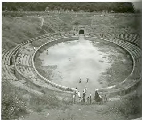
5.31 The amphitheater, Pompeii, ca. 80 BCE. This oval-shaped arena was used for the gladiatorial contests of which the Romans were exceedingly fond. Part of its seating is supported on arched construction and part is built into rising ground.
