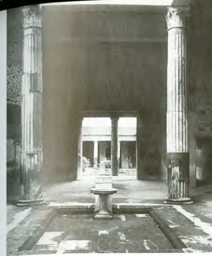
5-35 Atrium of the House of Venus in the Shell, Pompeii, 2nd century BCE. The roof has been restored to give an idea of the original space and light quality. Water running off the roof collected in the impluvium at the center of the atrium. Fresco painting can be seen at the left. The opening in the center led to the garden peristyle. Notice the opus incertum stonework facing of the walls.
