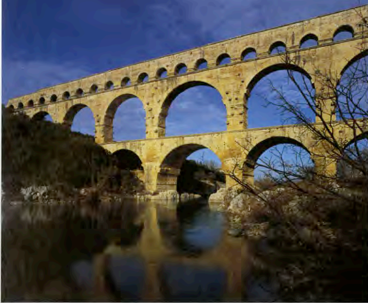
5-4 Pont du Gard, Nîmes, 20–16 BCE. The water channel (aqueduct) runs along the uppermost level, which maintains a constant incline to carry the water, through the pull of gravity, from nearby mountains into the city of Nîmes. Aqueducts ran along the contours of the land whenever possible, but when a valley had to be crossed, as here, Roman engineers used arches to span the gap. Projecting stones and inset holes were used for bracing the wooden centering, or scaffolds, needed to erect the arches, and they were left in the finished work in case repairs were ever required. This aqueduct has long been severed, so the Pont du Gard no longer carries water.
