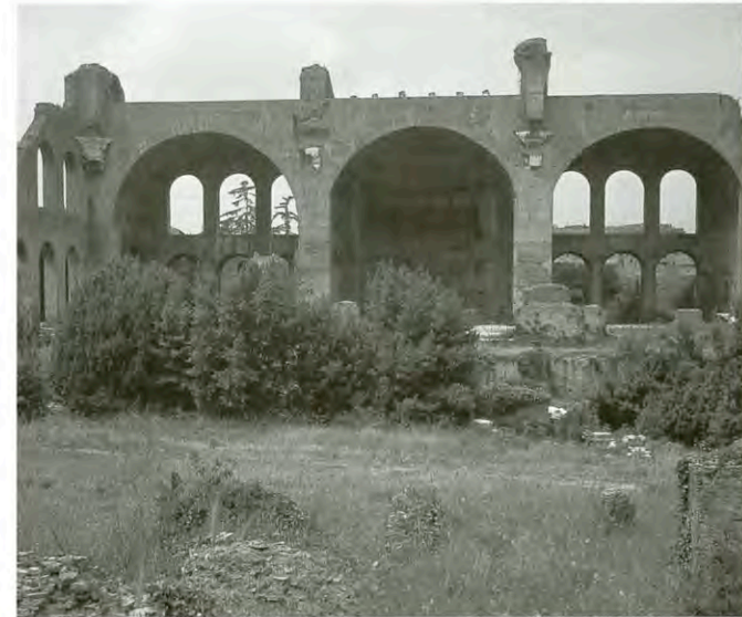
5.25 (right) Basilica Nova, Rome, 307–15 CE. Although the groin vaults have collapsed, one set of barrel vaults remains. Astride each bay, the haunches of the groin vaults rise above the parapet. The columns that stood below them were only ornamental.
