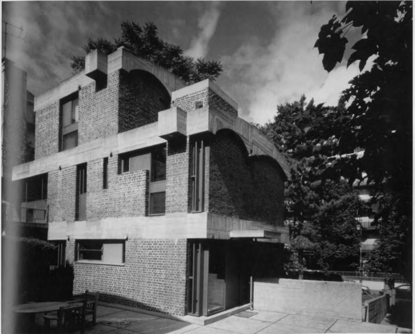
(Below) Maisons Jaoul, Neuilly-sur-Seine, France. Le Corbusier, 1955. A new acceptance of natural materials and traditional form: brick and wood with 'Catalan' vaults.
