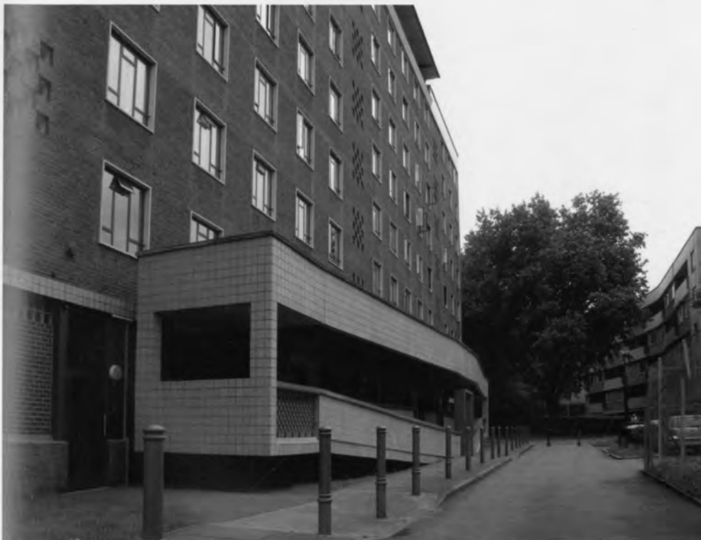
Spa Green Estate, London, UK. Berthold Lubetkin, 1949. An early example of 'box frame' construction but clad in brick and tiles.
