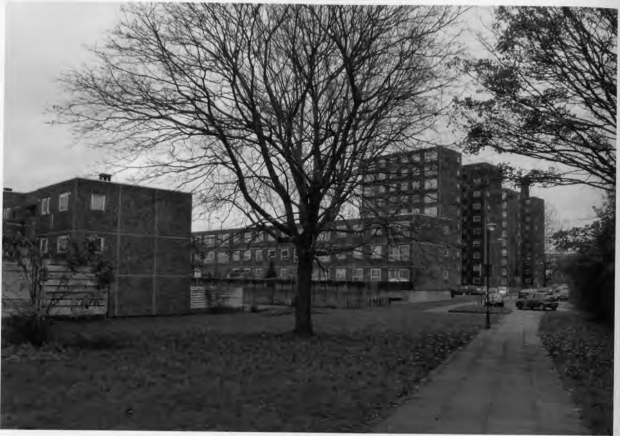
Morris Walk Estate, London. Martin Richardson, 1966. The Danish Larsen-Nielsen system adapted to the British preference for mixed developments.
