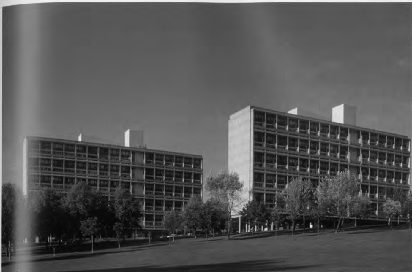
Alton West, Roehampton, UK. London County Council Architect, 1958. Slab blocks obviously influenced by Le Corbusier's Unité, but on a smaller scale.
