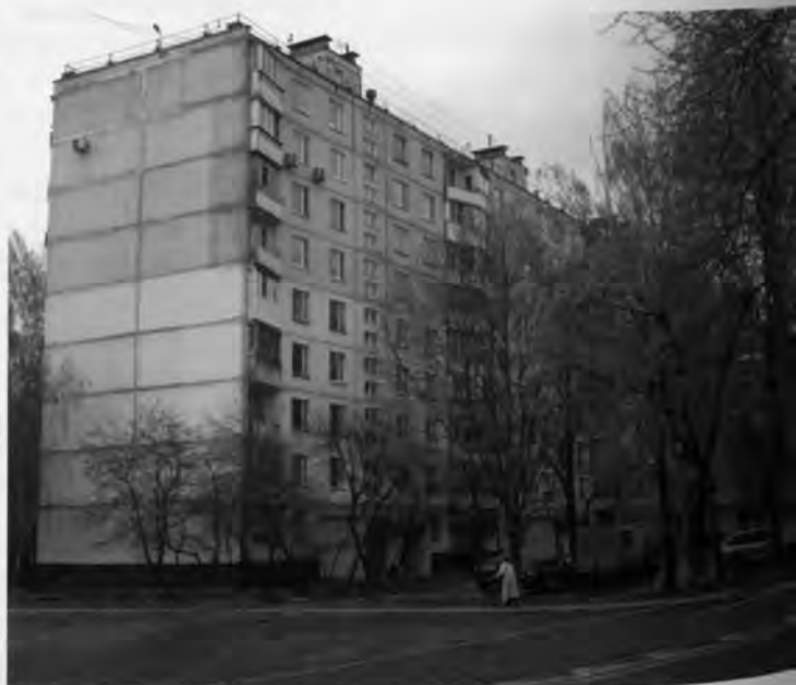
1960s apartments in Belyayevo, Moscow. Later, nine-storey versions of the K-7. Construction was notoriously shoddy.
