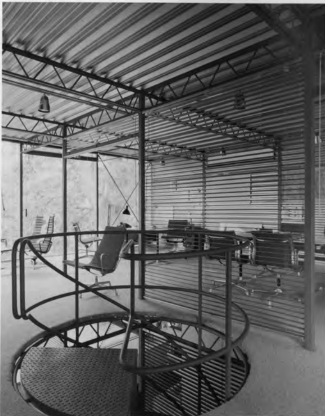
Hopkins House, London, UK. Michael Hopkins, 1976. The architect's own house, a homage to the Eames House in California of thirty years earlier.
