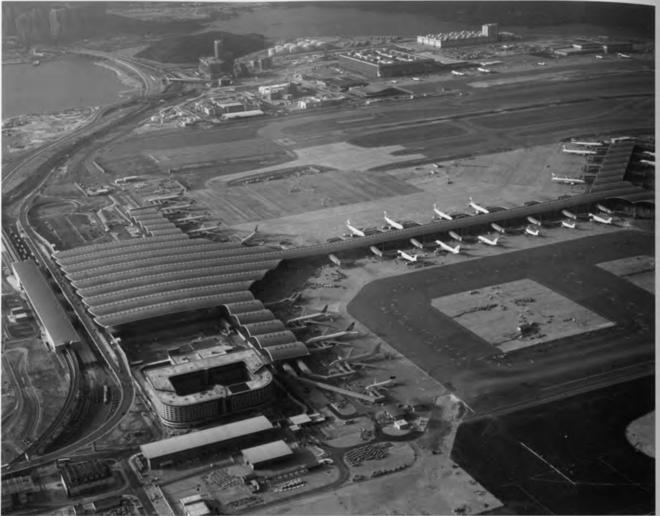
Chek Lap Kok Airport, Hong Kong, China. Norman Foster, 1998. The design principles of Stansted applied at a much larger scale on an artificially extended island.
