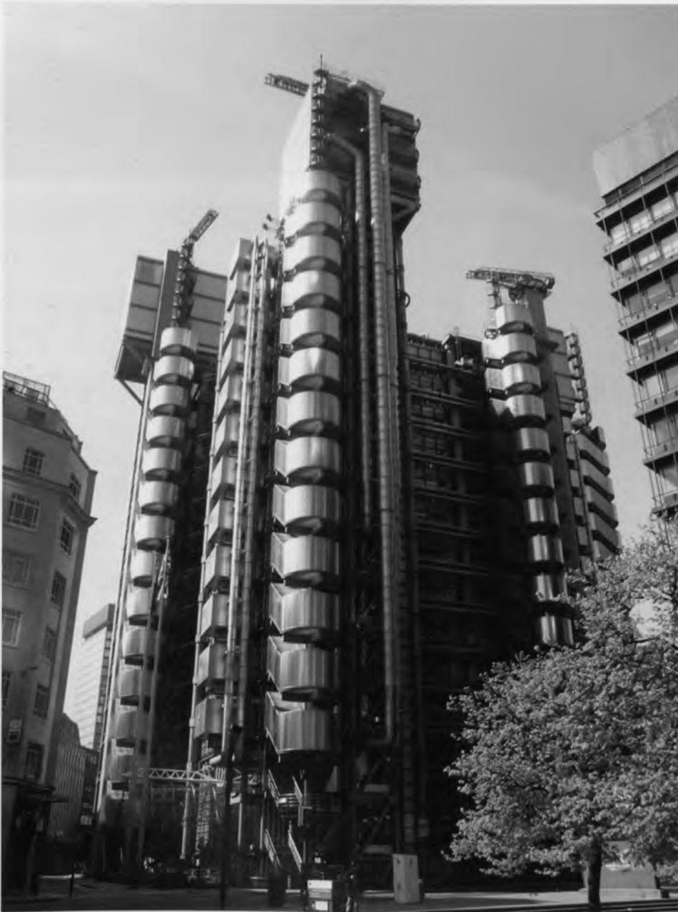
(Left) Lloyd's of London, London, UK. Richard Rogers, 1986. A complicated exterior makes possible a simple multi-storey 'omniplatz'.
