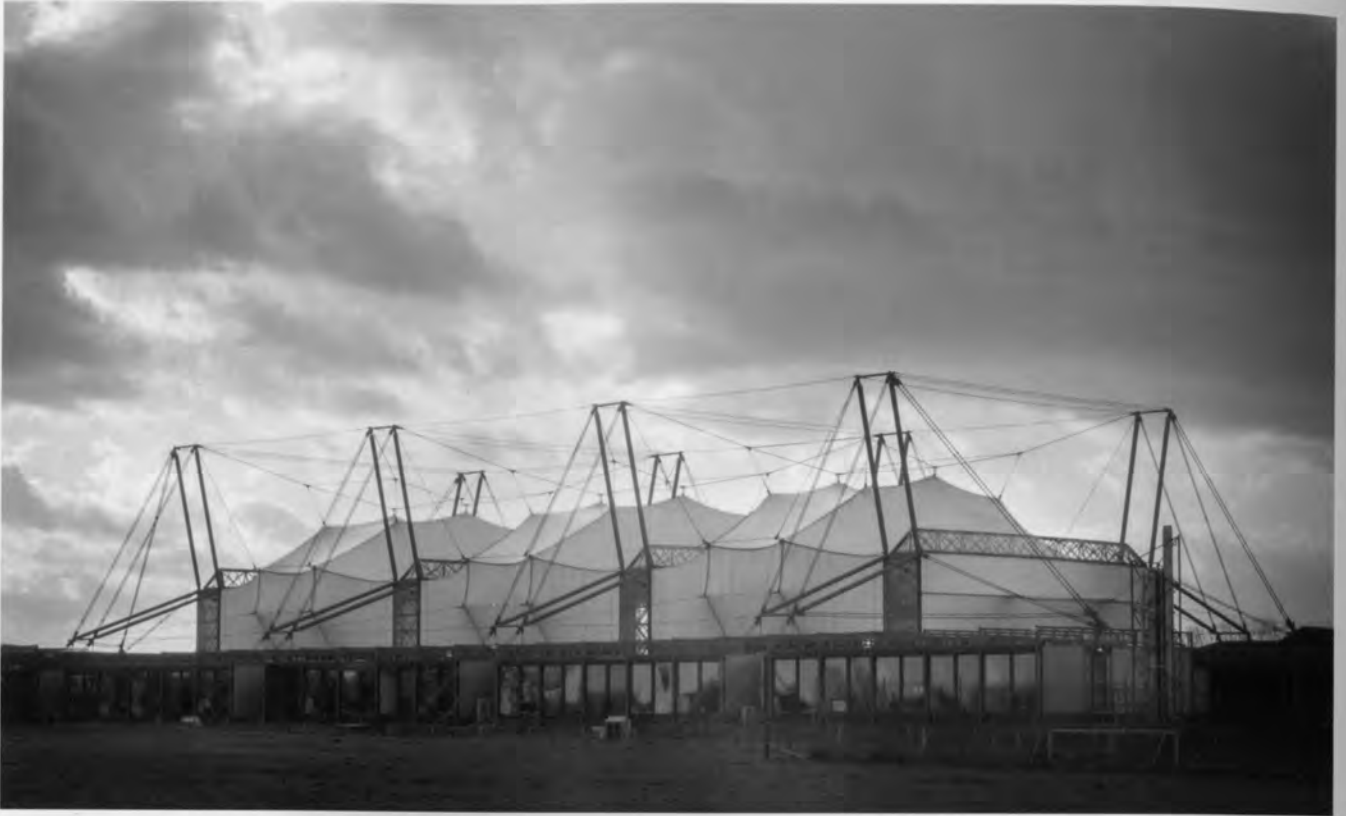
(Above) Schlumberger Research Centre, Cambridge, UK. Michael Hopkins, 1985. A tent like a circus big top covers a winter garden at one end and a drilling test rig at the other.
