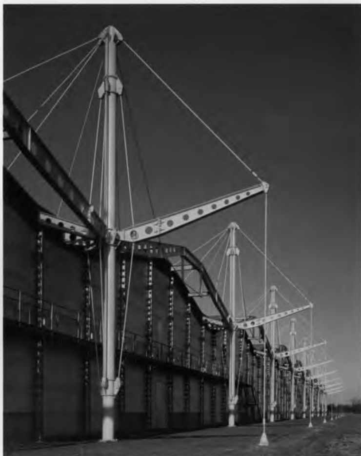
(Below) Renault Distribution Centre, Swindon, Wiltshire, UK. Norman Foster, 1982. Gothic High Tech: masts are anchored to the ground like reverse flying buttresses.
