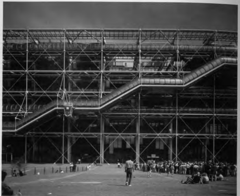
Centre Pompidou, Paris, France. Renzo Piano and Richard Rogers, 1977. Football pitches of flexible, fully serviced space created by an ingenious tensioned structure.
