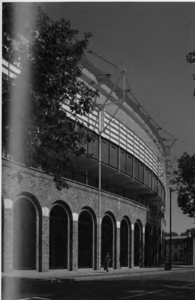
(Above) Glyndebourne opera house, Sussex, UK. Michael Hopkins, 1994. The High Tech doctrine of truth to materials still applies. Brick arcades are genuinely loadbearing.
