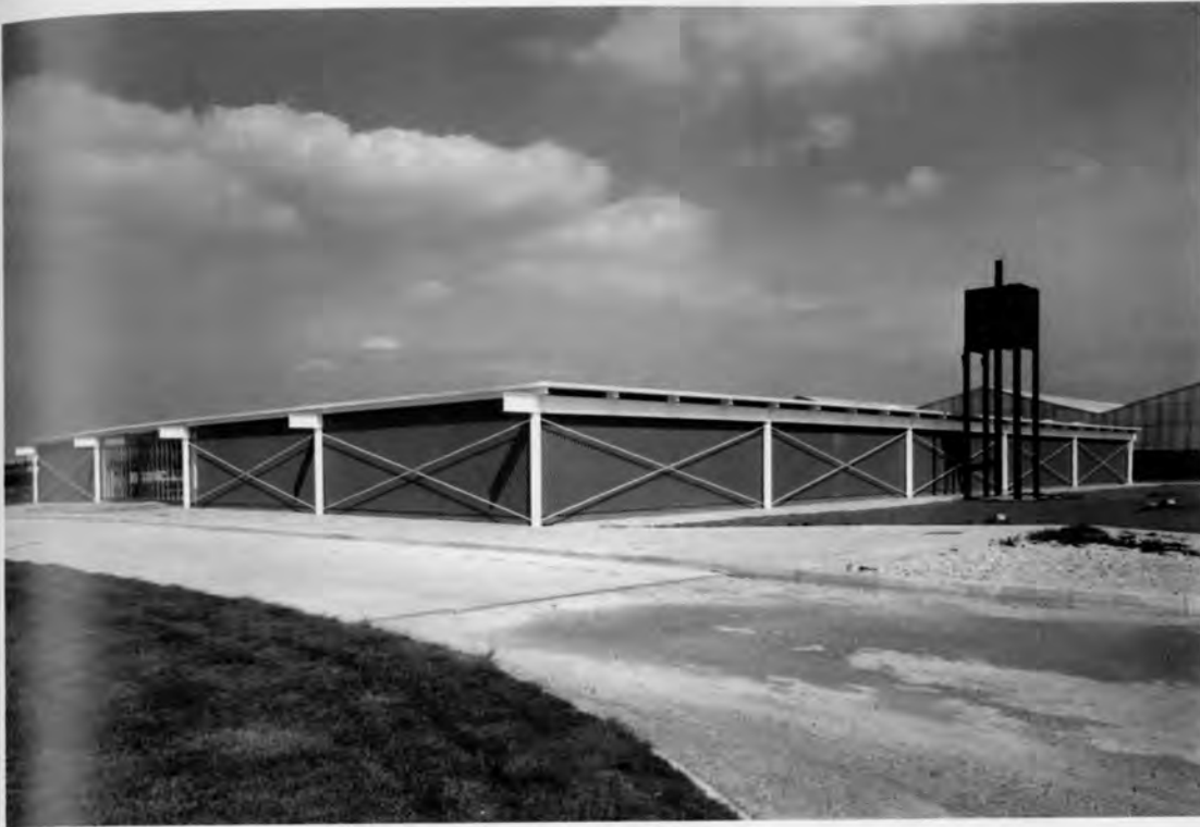
Reliance Controls Factory, Swindon, Wiltshire, UK. Team 4, 1967. Diagonal bracing, not strictly necessary in every bay, takes the basically Miesian structure in a new direction.
