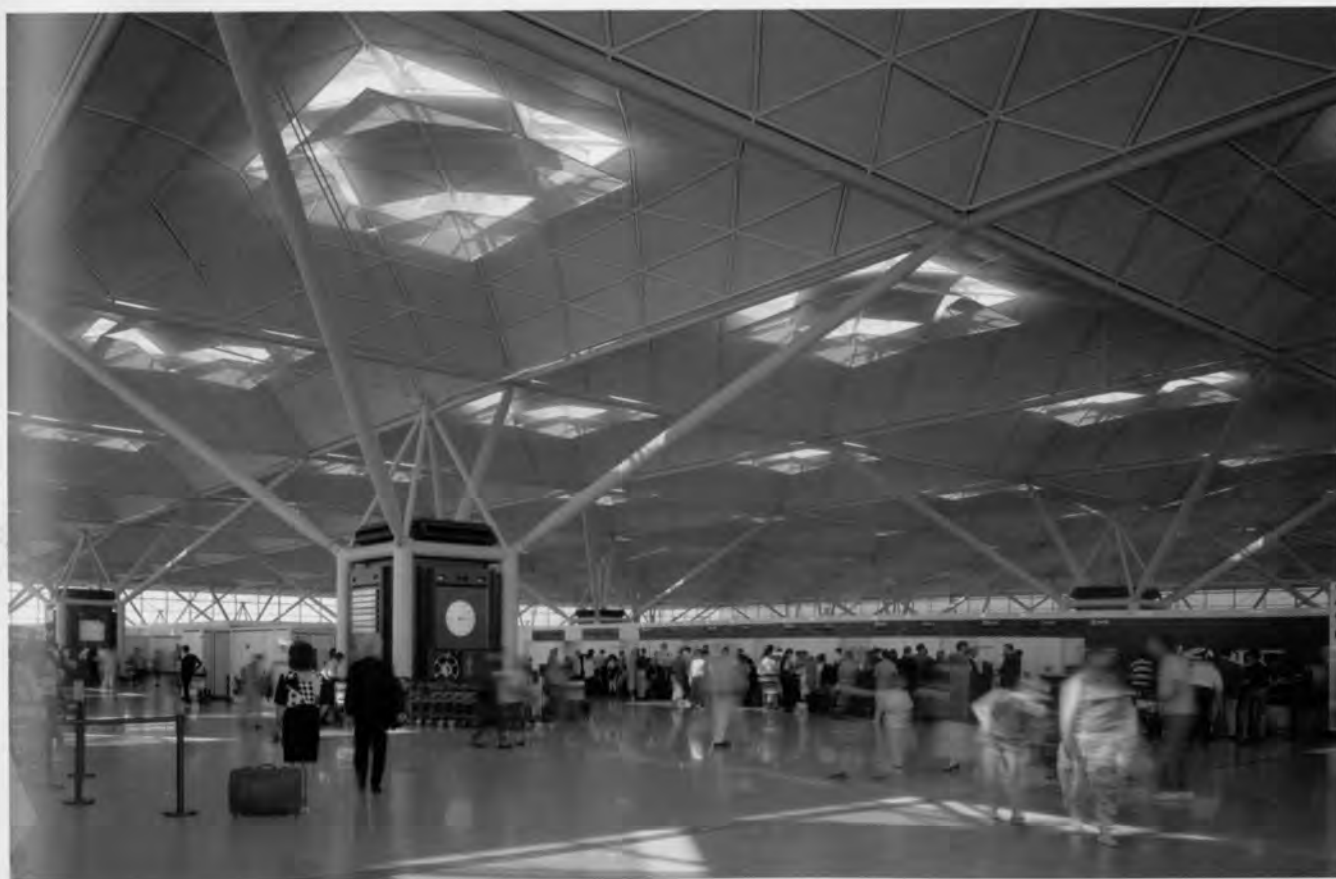
London Stansted Airport, Essex, UK. Norman Foster, 1991. A high, day-lit space, roofed by square domes and cleared of the clutter of mechanical and electrical services.
