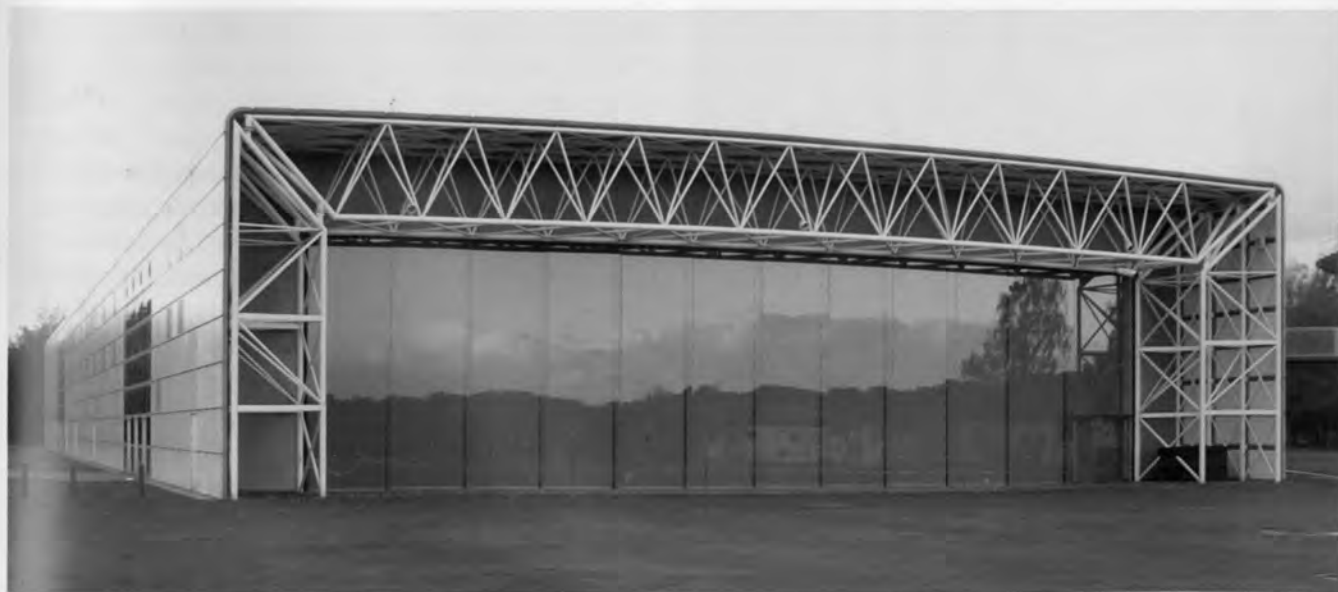
Sainsbury Centre exterior. Structure and services wrap around the space; factory-like in appearance as well as concept.
