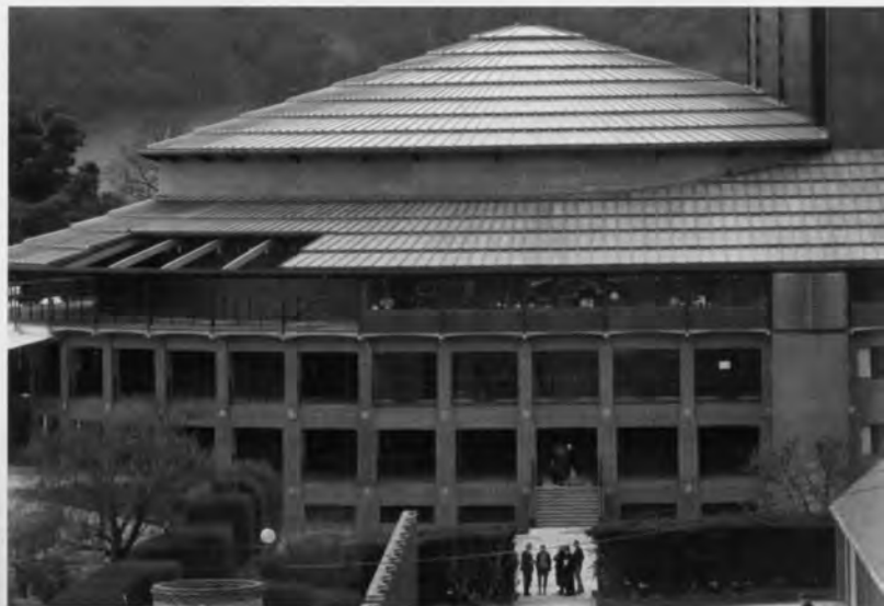
(Above) Glyndebourne opera house, Sussex, UK. Michael Hopkins, 1994. The High Tech doctrine of truth to materials still applies. Brick arcades are genuinely loadbearing.
