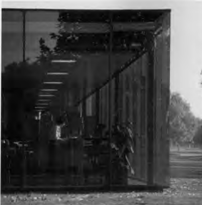
IBM Headquarters, Cosham, Hampshire, UK. Norman Foster, 1971. Utter simplicity: open planned and flat roofed with external walls of full-height glass in neoprene gaskets.
