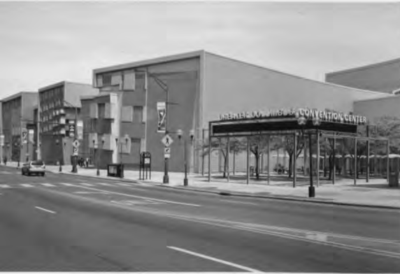
Greater Columbus Convention Center, Ohio, USA. Peter Eisenman, 1993. The street front reveals the ends of train-like roofs, though the space below is a simple hall.
