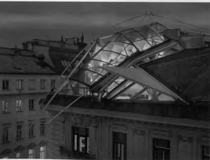
(Above) Rooftop remodelling, Falkestrasse, Vienna, Austria. Coop Himmelb(l)au, 1988. The insect-like form might have been the result of a blind drawing exercise.
