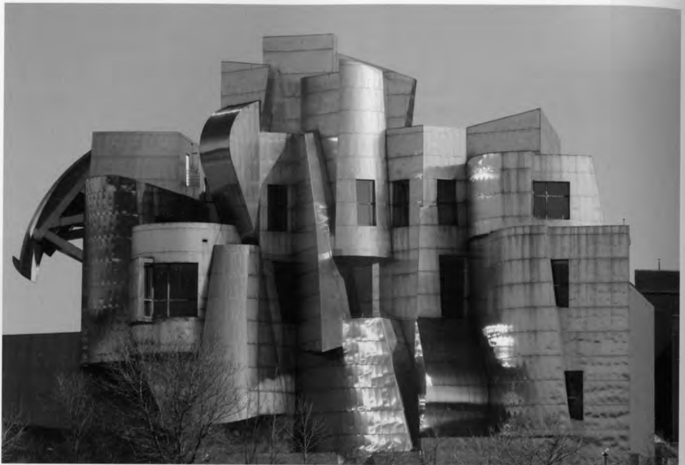
Weisman Art Museum, University of Minnesota, Minnesota, USA. Frank Gehry, 1993. Deconstructed to an extreme degree, like a Cubist sculpture.
