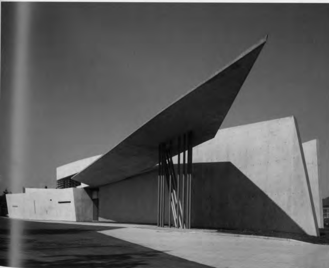
Vitra Fire Station, Weil am Rhein, Germany. Zaha Hadid, 1993. Reinforced concrete stretched to the structural limit in Zaha Hadid's first important building.
