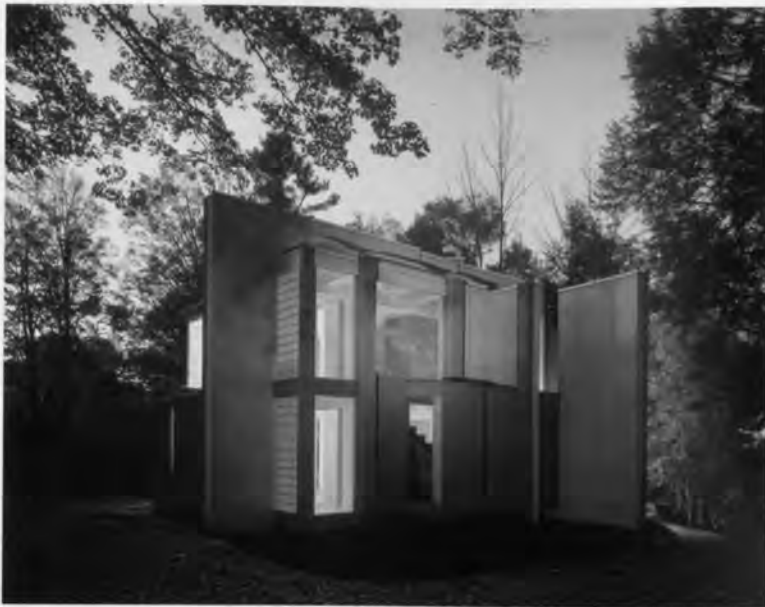
House VI, Cornwall, Connecticut, USA. Peter Eisenman, 1973. The composition, including an upside-down staircase, is the outcome of a sequence of formal transformations.
