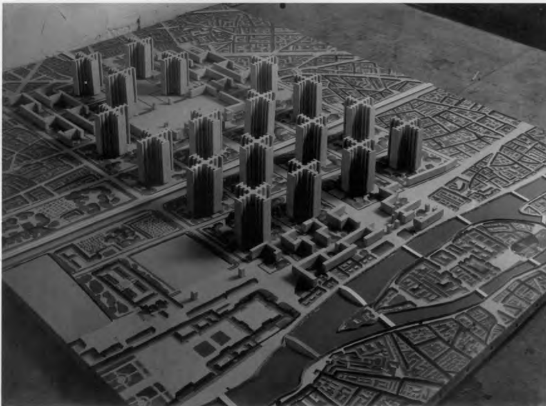
Plan Voisin project for Paris. Le Corbusier, 1922. A shining new city was envisaged, but also the destruction of one of Paris's most loved districts.
